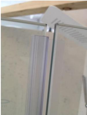
14. Install waterproofing gasket on bottom of door with rubber mallet.
