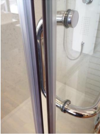
12. To adjust door seal, use the angled support arms to make slight adjustments in the angle of glass.
